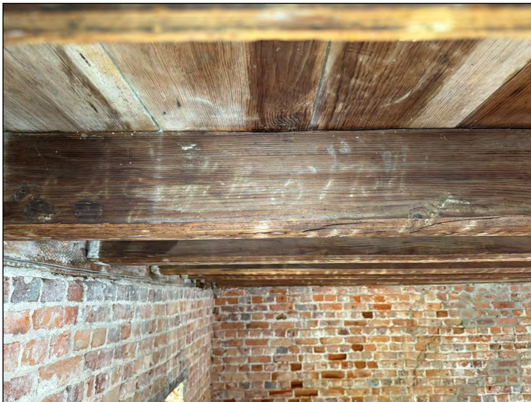
Hall, ceiling detail, “August th5 1754” [or 1734?].
