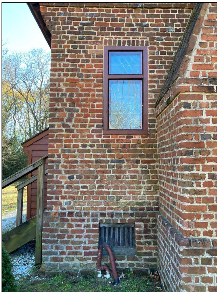
North side elevation, original sized window openings
