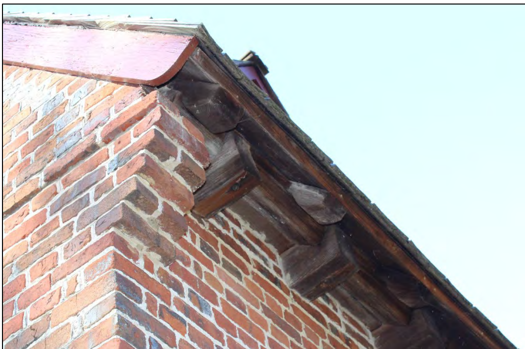
Cornice detail, SE corner, December 2023
