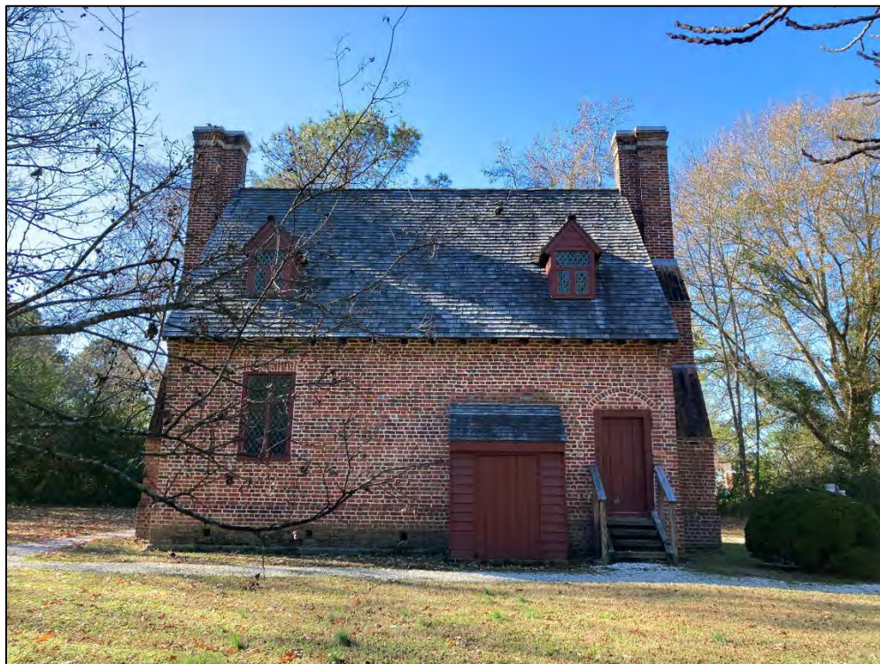
Rear elevation, December 2023.
