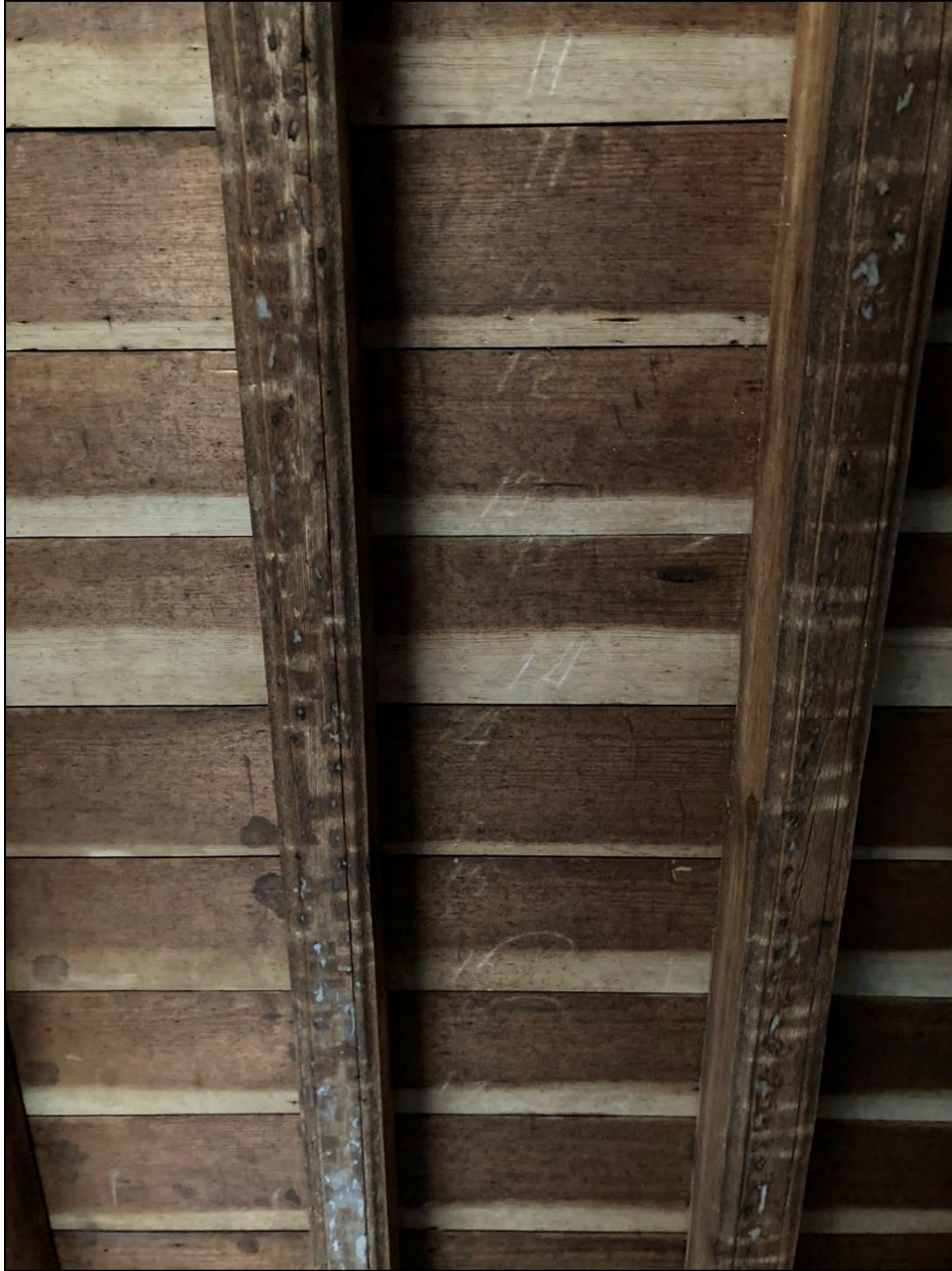
Hall, ceiling detail, exposed joists and numbered floorboards. December 2023.
