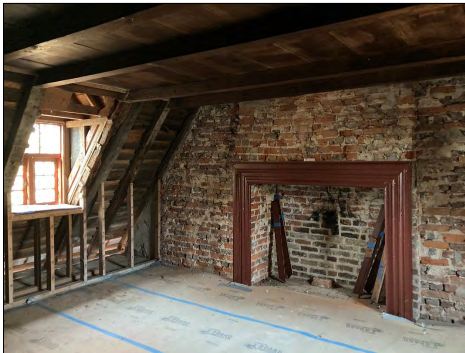
Second floor, parlor chamber. May 2024.
