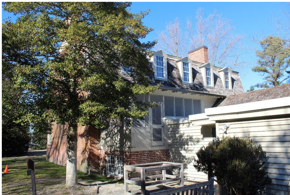
Figure 7: Rear porch on original block
