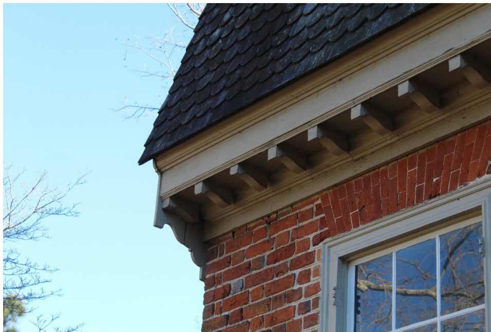
Figure 5: Detail of roof cornice on facade
