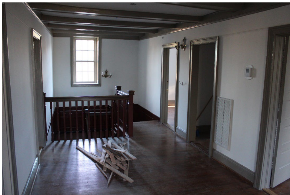
Figure 15: Second story, central hallway looking towards rear
