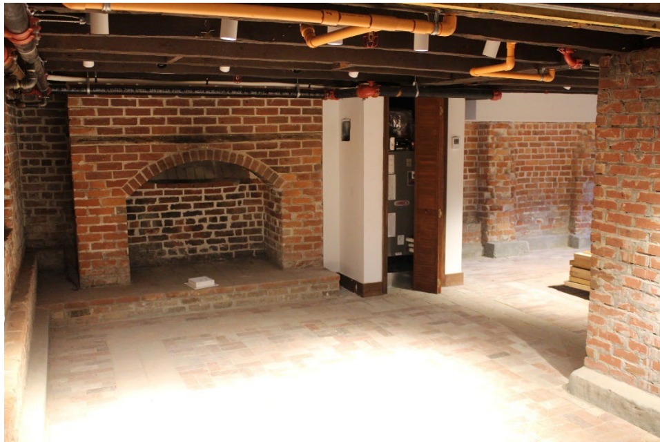
Figure 20: Basement, cooking hearth under southwest room
