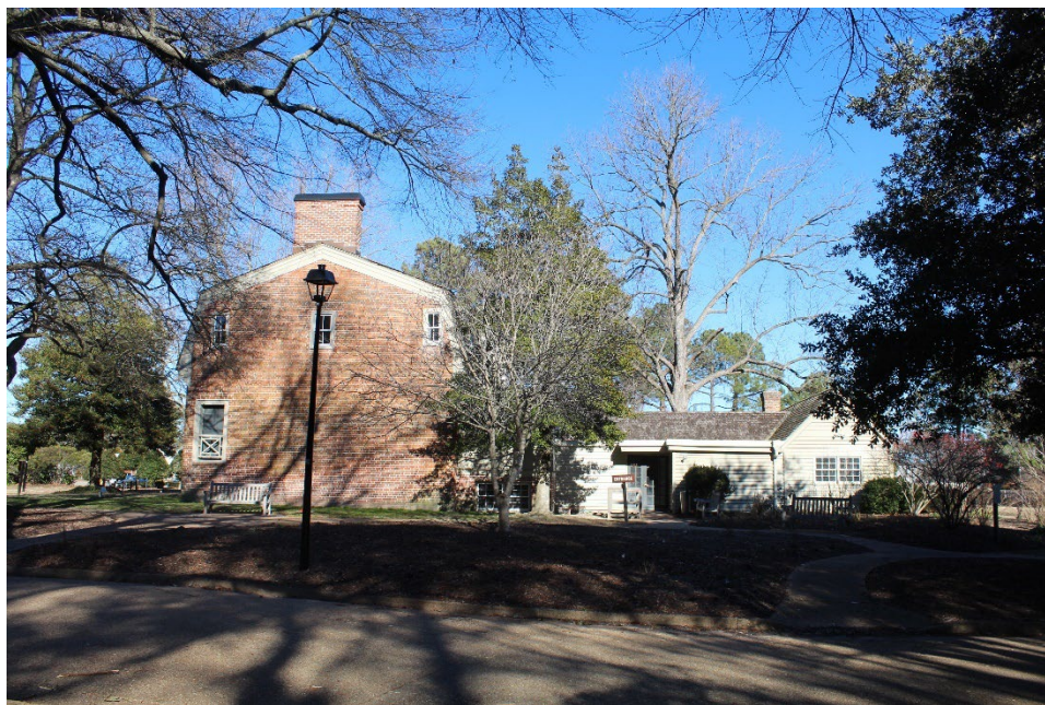
Figure 9: West side with rear addition
