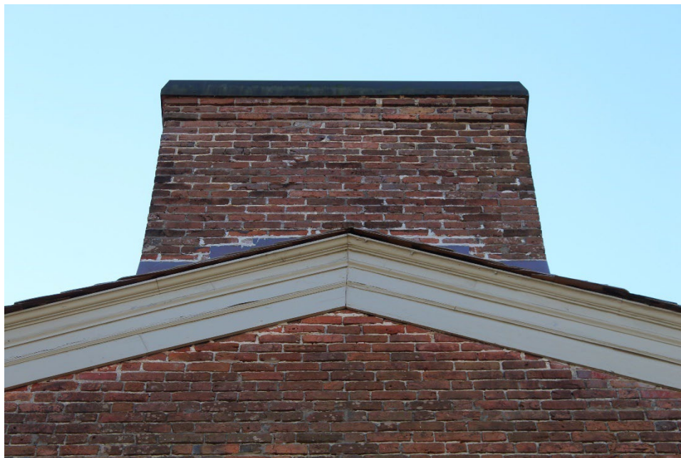
Figure 6: Detail of chimney and raking cornice
