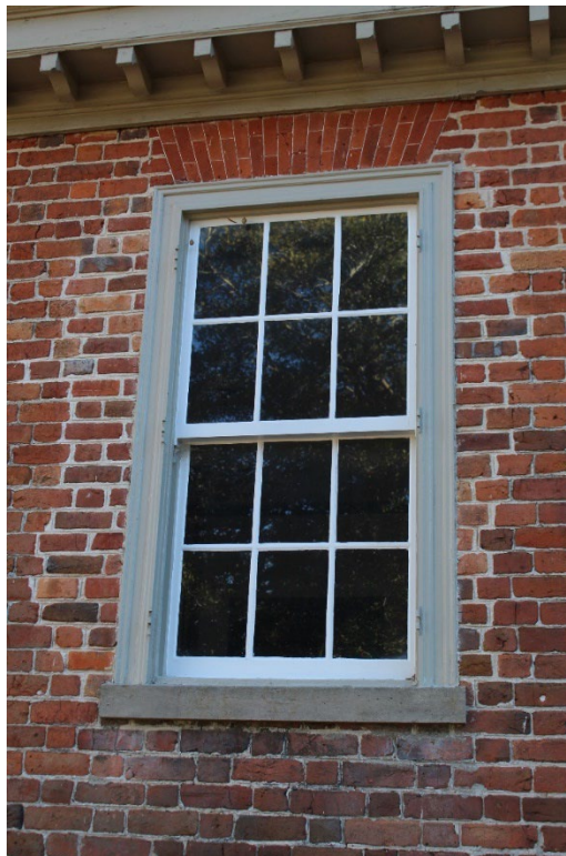
Figure 4: Detail of window opening on facade
