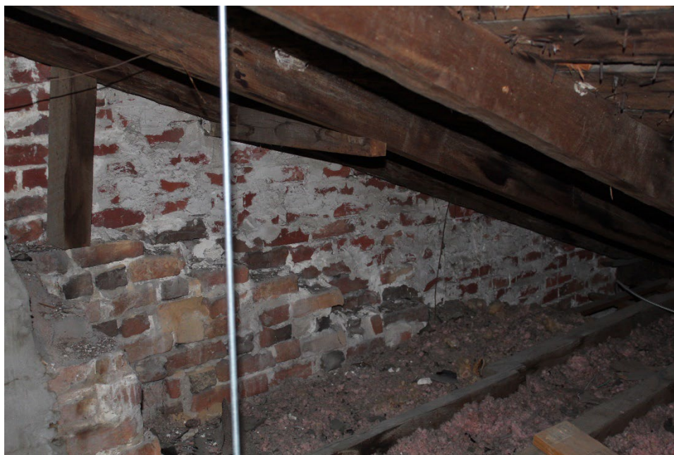
Figure 21: Relic brickwork in attic revealing lift of gambrel roof
