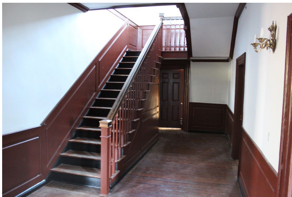
Figure 10: First story central passage looking towards rear
