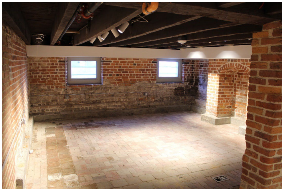
Figure 19: Basement, room under east side of house
