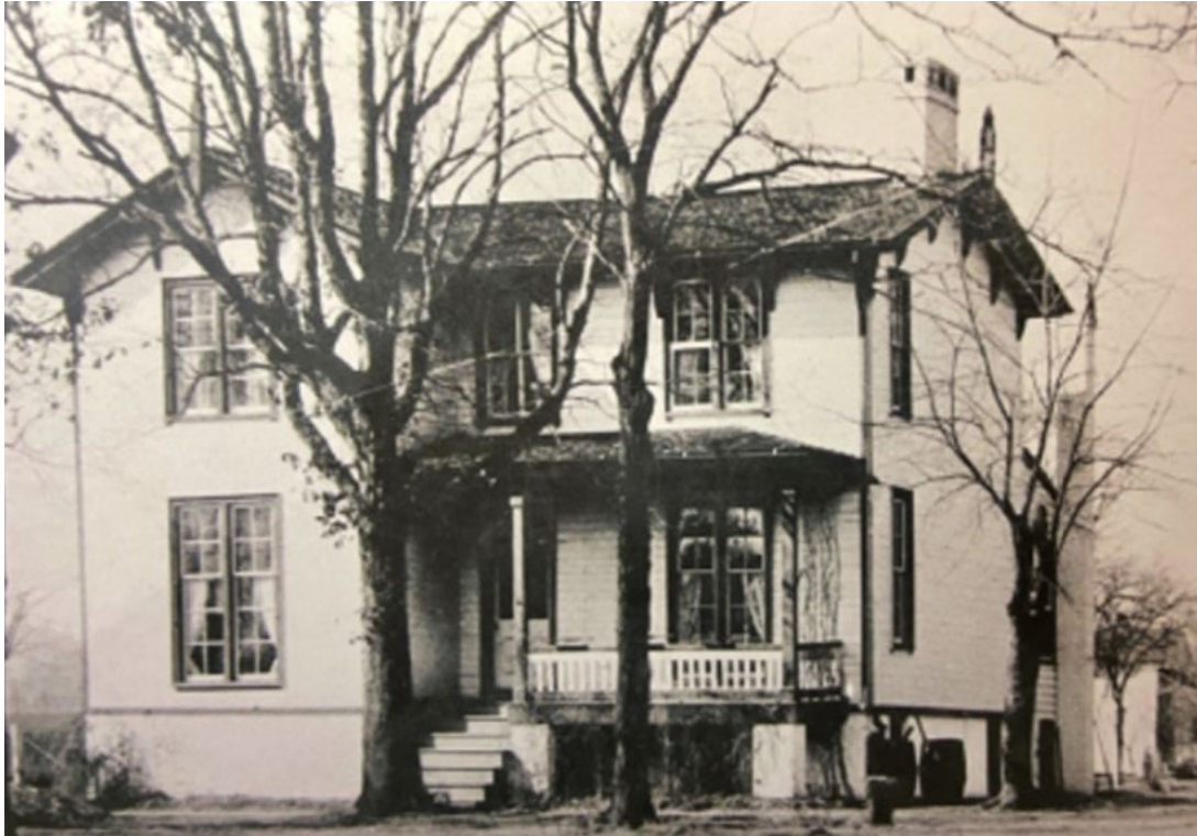
Figure 2: Undated photograph of the façade of the keeper's lodge. Note brackets under the cornice and tall first story windows. (Source: Ivy Hill Cemetery)
