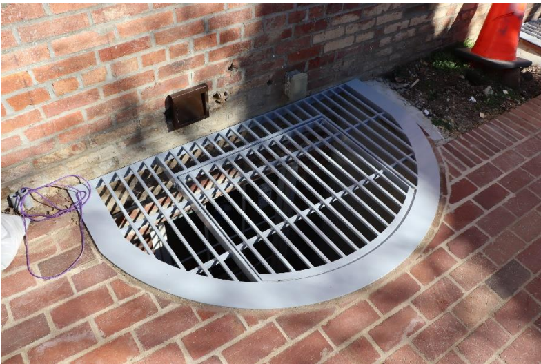
2024: South wall of main block, new basement windows and window wells
