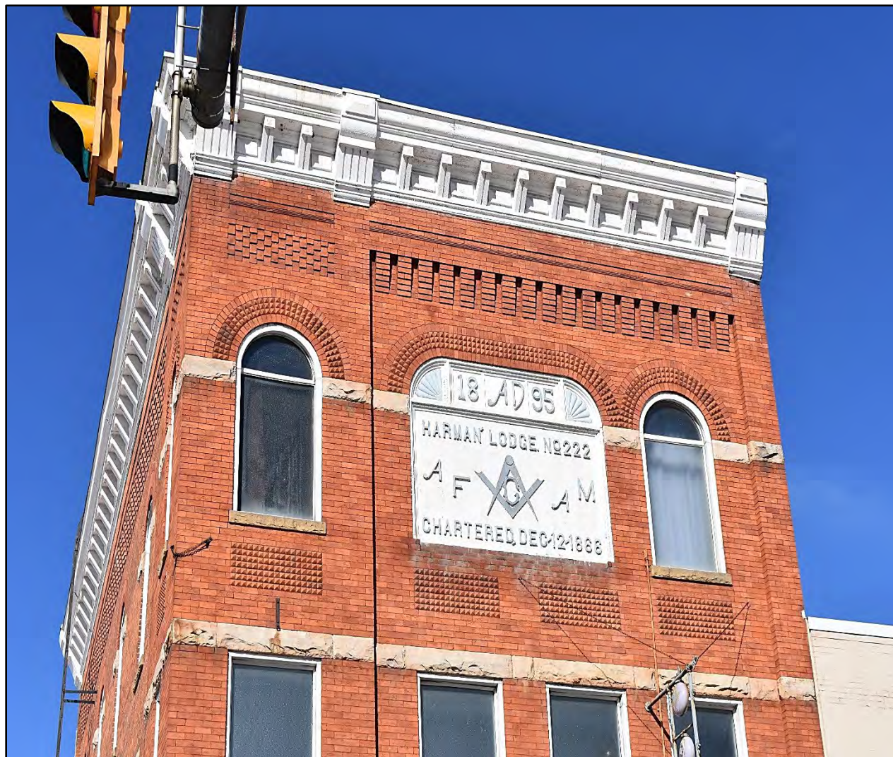
Figure 2. Detail of Harman Lodge No. 222 Showing Plaque on Front of Building and Decorative Brick Detailing.
