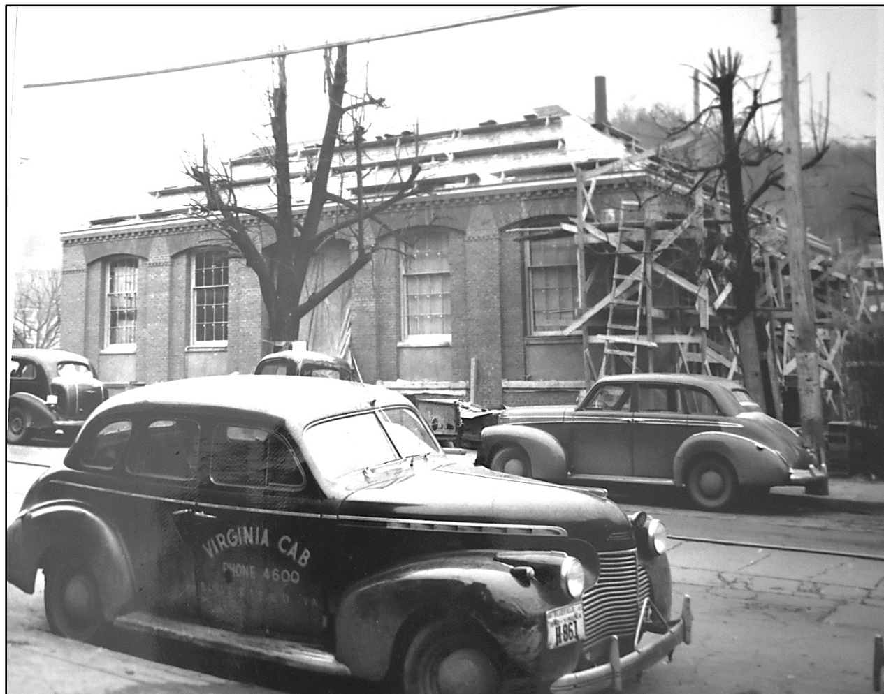
Figure 9. Bluefield Post Office Construction Nearing Completion, January 19, 1941. Source: Lisa Byrd.
