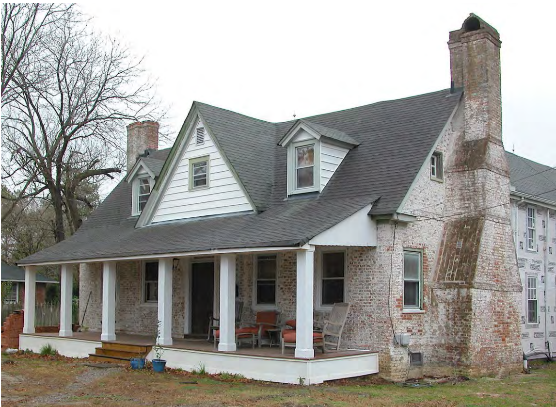
Fox Hall Before Restoration
