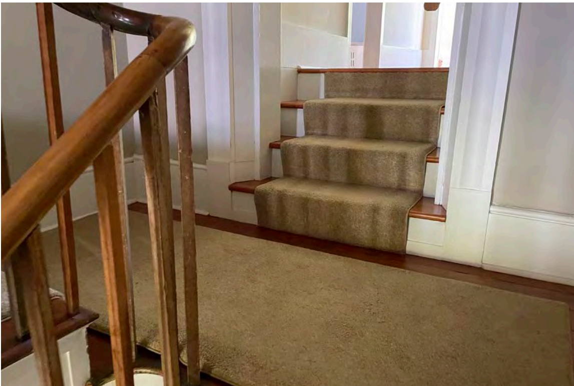
PHOTO 28 DATE: May 2024 DESCRIPTION: Second Floor stair detail into rear addition.
