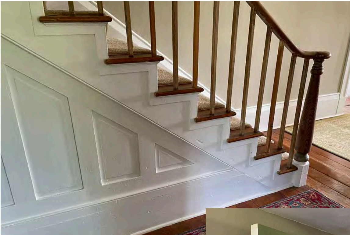
PHOTO 13 DATE: May 2024 DESCRIPTION: First Floor stair detail.
