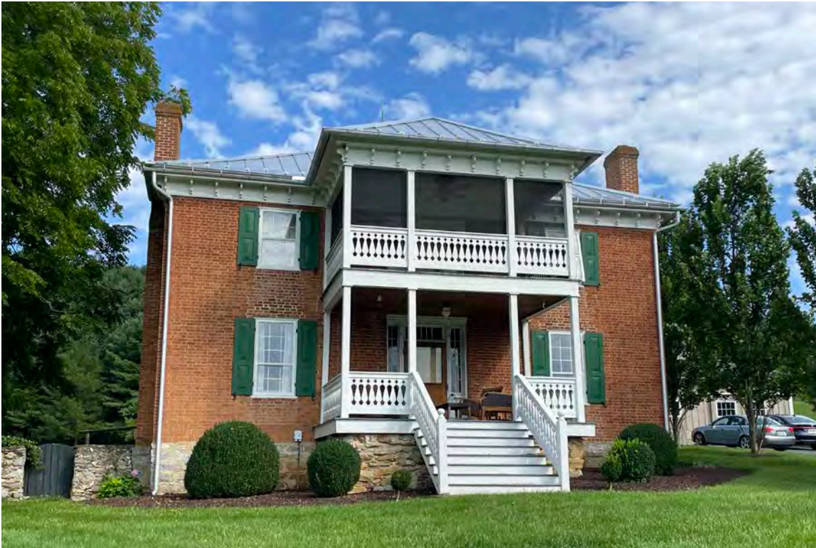
PHOTO 5 DATE: May 2024 DESCRIPTION: Front (east) elevation
