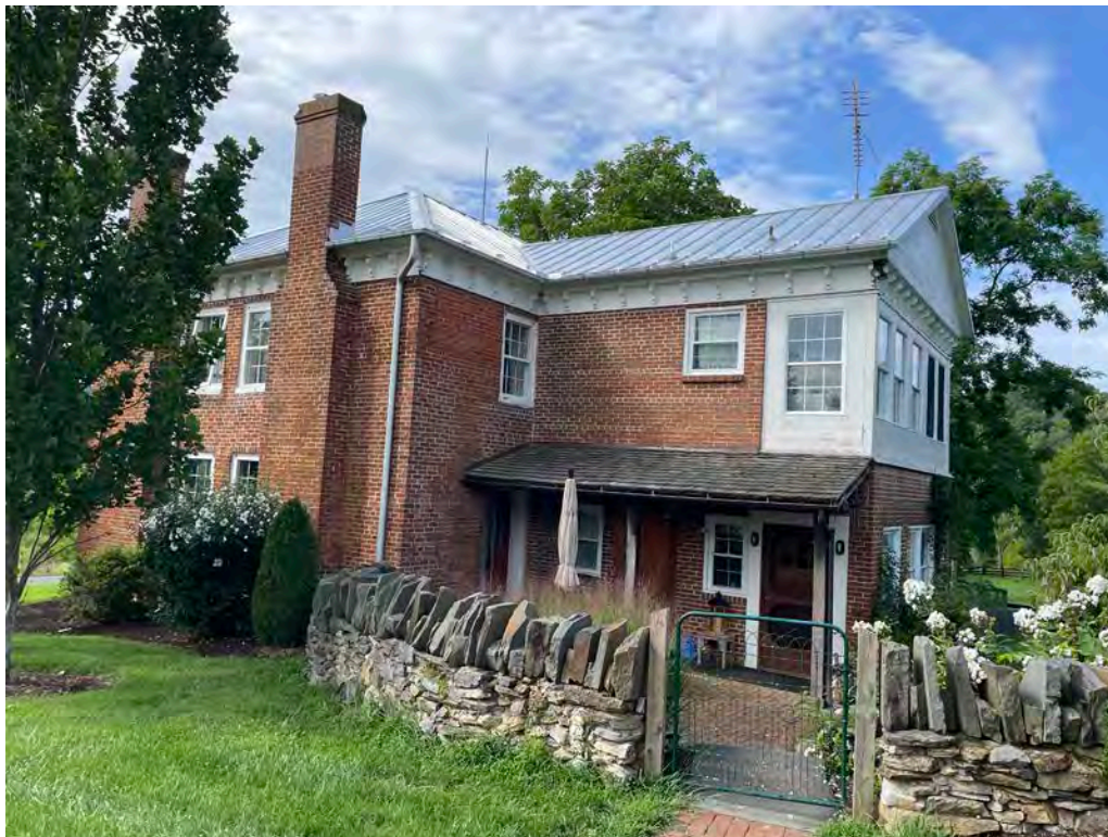
PHOTO 6 DATE: May 2024 DESCRIPTION: North elevation
