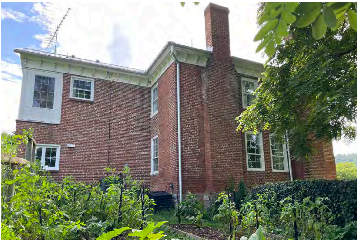
PHOTO 8 DATE: May 2024 DESCRIPTION: South elevation
