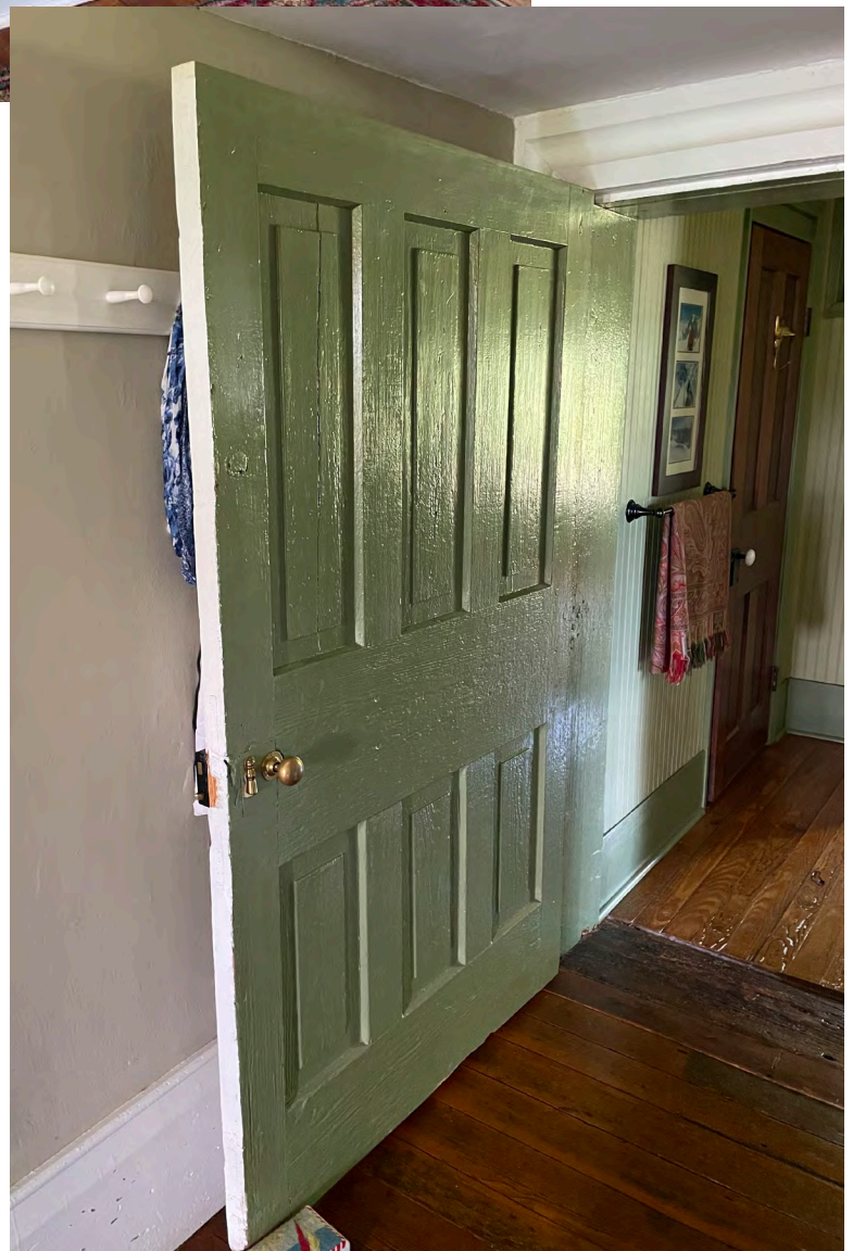
PHOTO 14 DATE: May 2024 DESCRIPTION: First Floor typical six-panel door.
