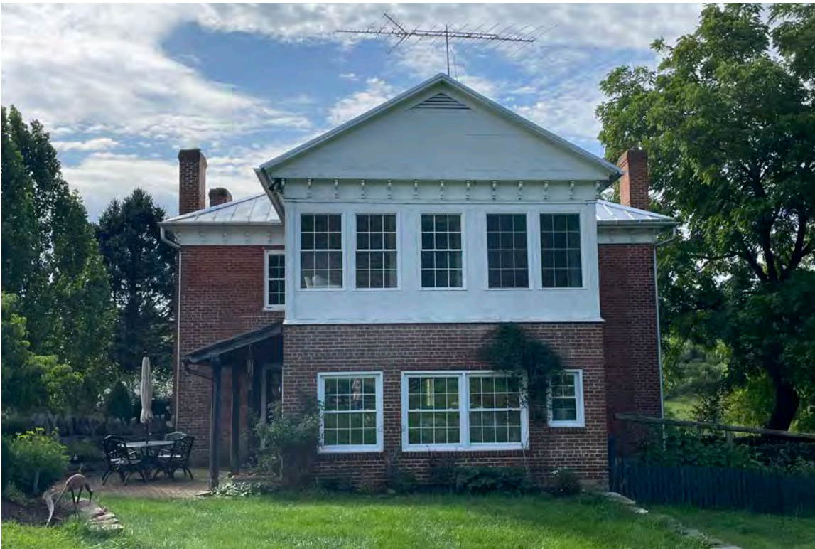
PHOTO 7 DATE: May 2024 DESCRIPTION: West elevation
