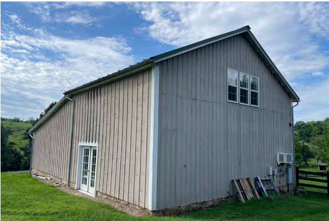
PHOTO 2 DATE: May 2024 DESCRIPTION: Outbuilding 1, Garage; north and east elevations.
