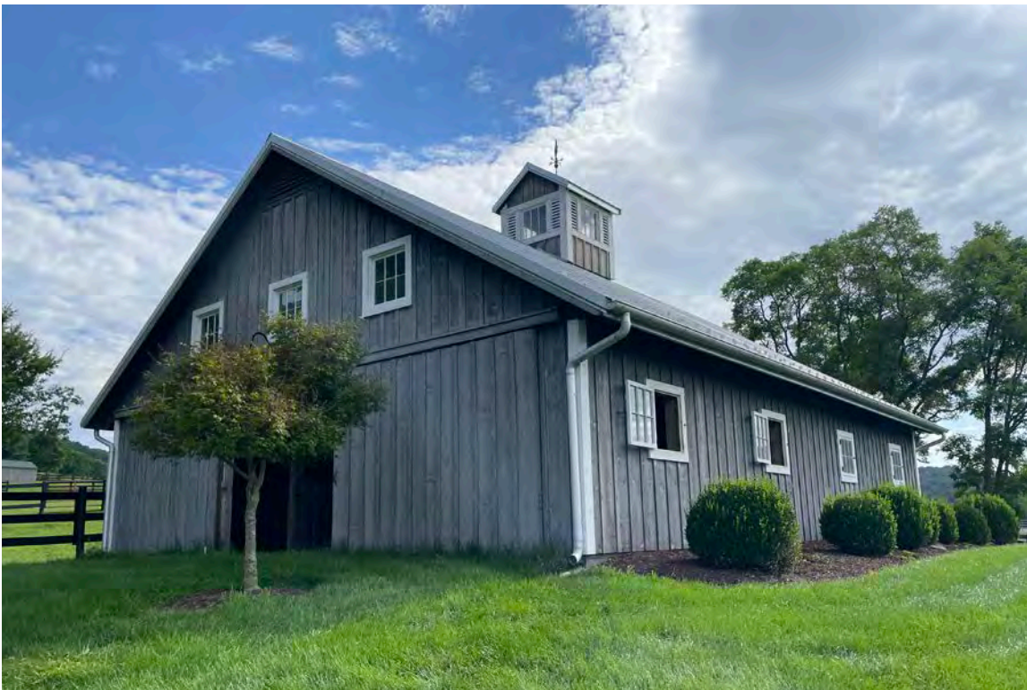
PHOTO 4 DATE: May 2024 DESCRIPTION: Outbuilding 3, Horse Barn
