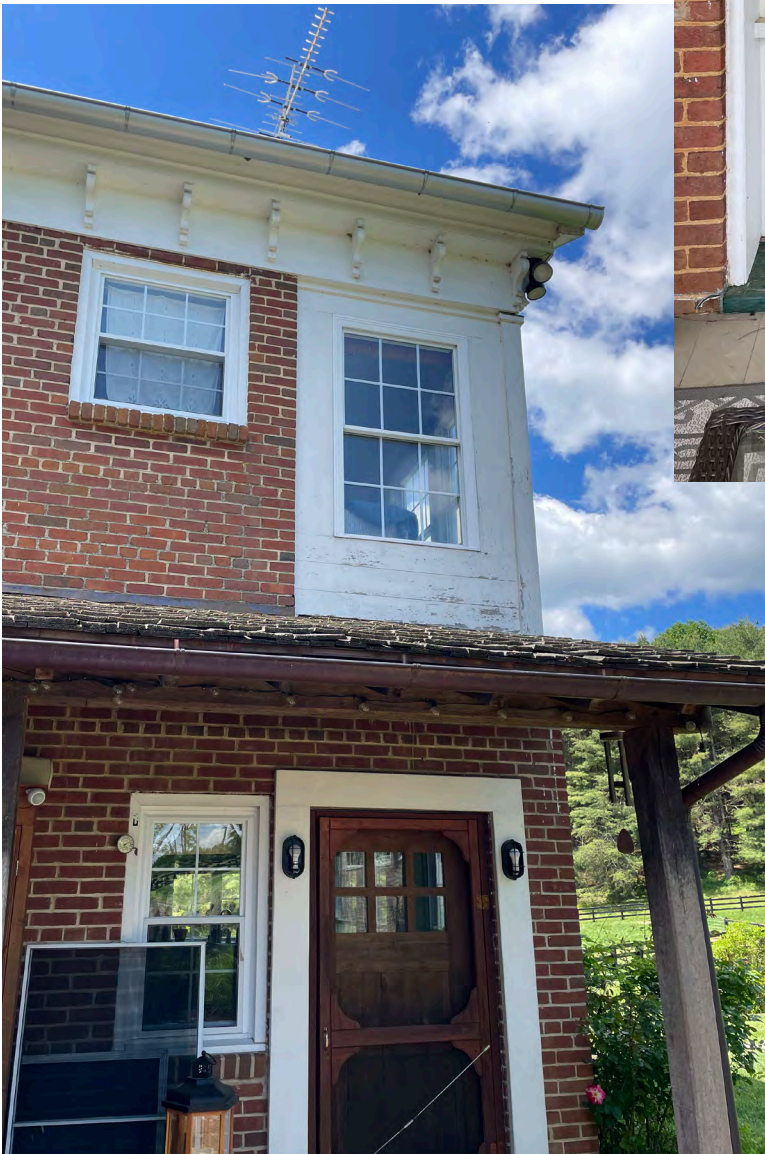
PHOTO 10 DATE: May 2024 DESCRIPTION: North elevation detail
