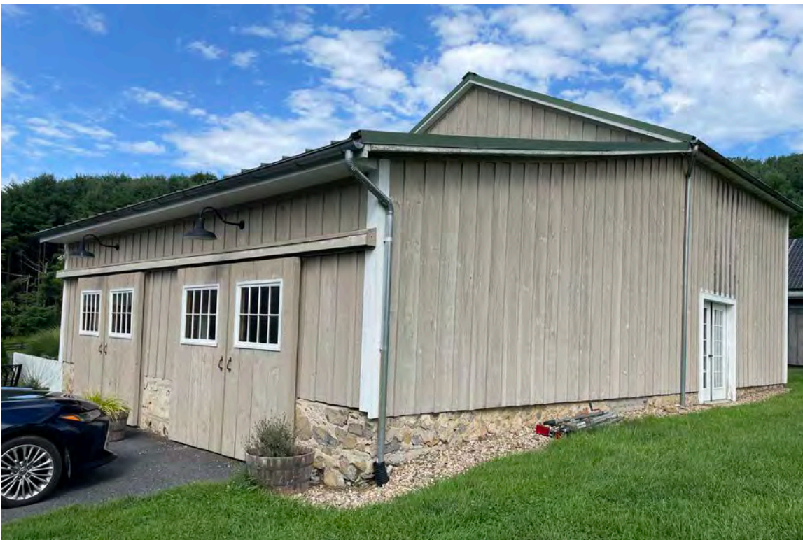
PHOTO 1 DATE: May 2024 DESCRIPTION: Outbuilding 1, Garage; south and east elevations.
