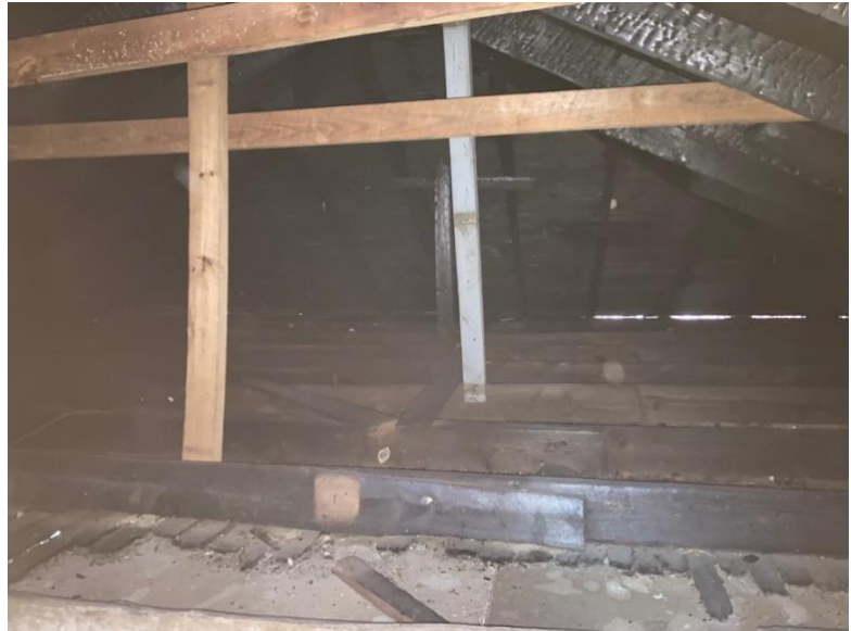
ATTIC, FACING EAST
