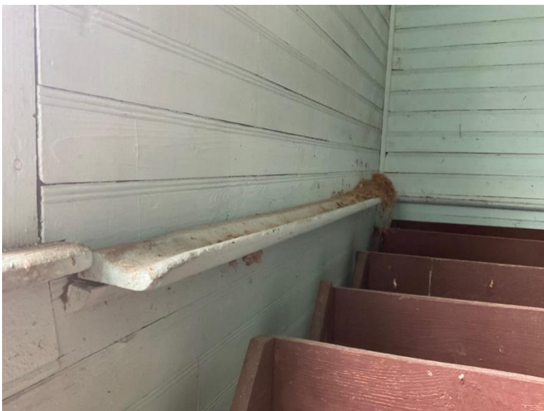
CHALK TRAY ON WEST WALL IN WEST CLASSROOM
