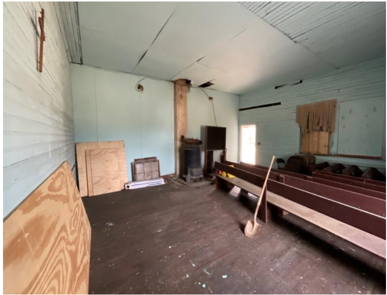
WEST CLASSROOM, FACING SOUTHEAST
