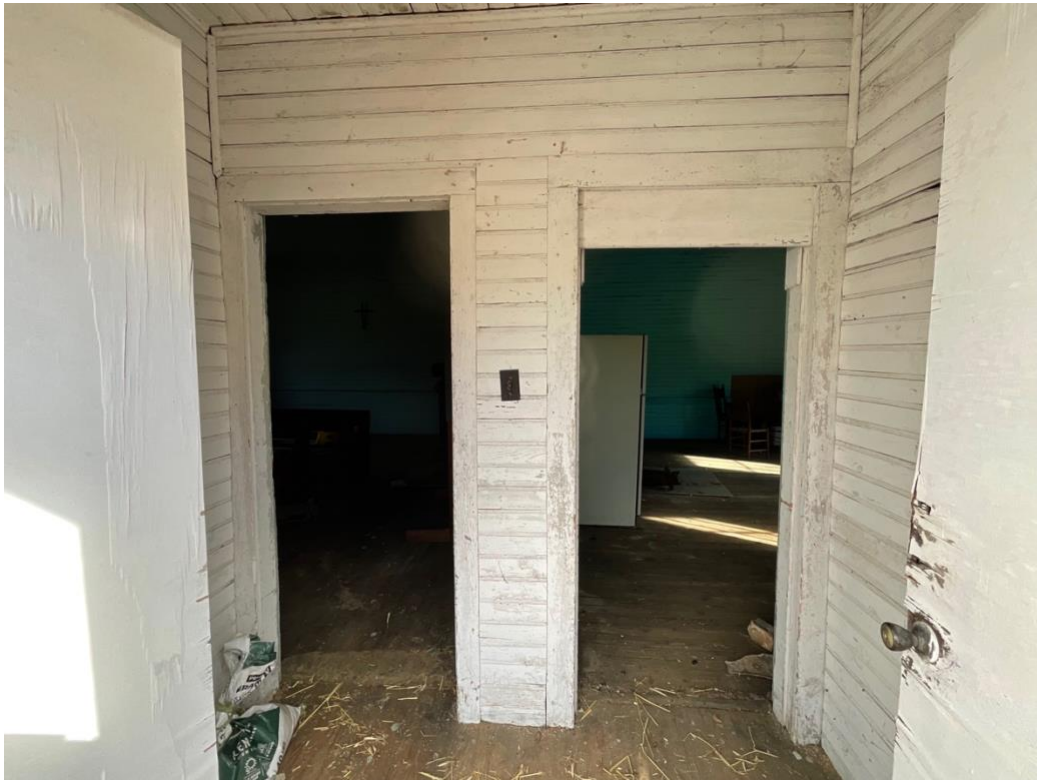
VESTIBULE, FACING NORTH TOWARDS CLASSROOM DOORS
