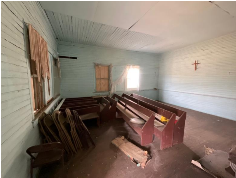
WEST CLASSROOM, FACING NORTHWEST
