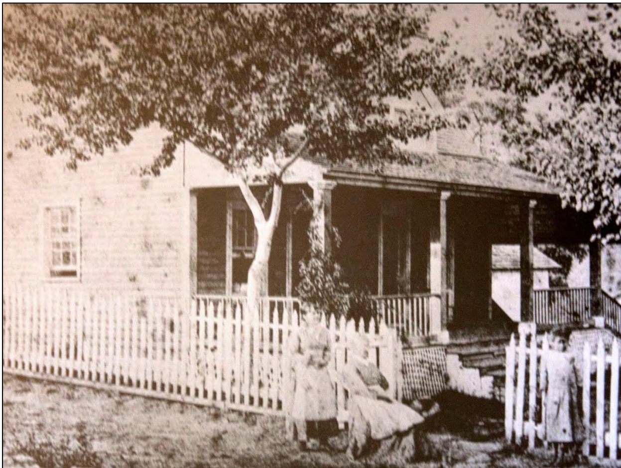
Figure 7. Photograph, c. 1875, showing the façade and west elevation of Drover's Rest (Special Collections, Fairfax County Public Library)
