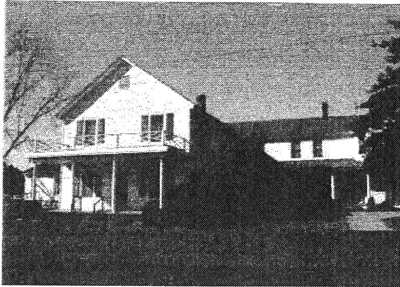
Figure 35: Williams Store and Wan Post Office (036-5033) South facade
