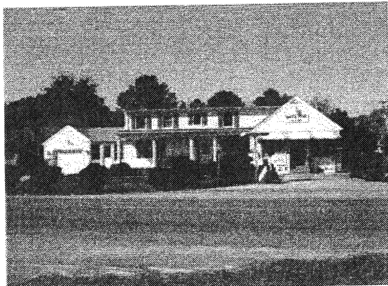
Figure 44: Bland's Store (036-5008) East façade
