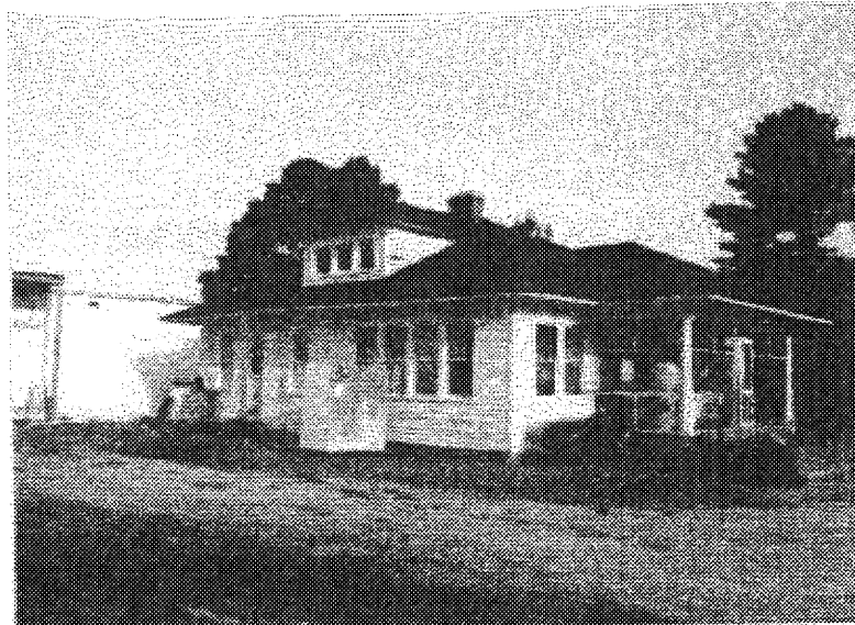
Figure 36: Poland's Store (036-5020) Southeast corner
