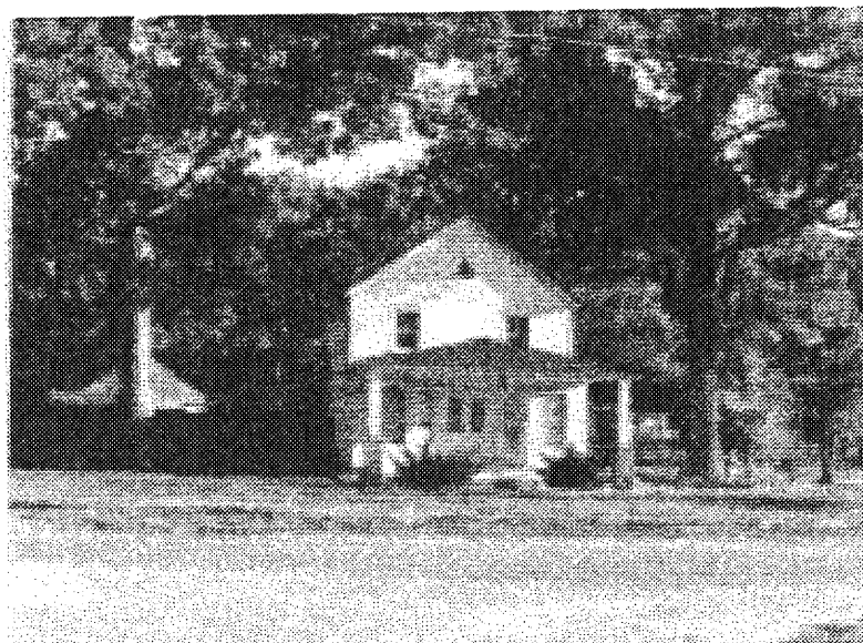
Figure 10: Pinero Store and Post Office (036-5014) West façade
