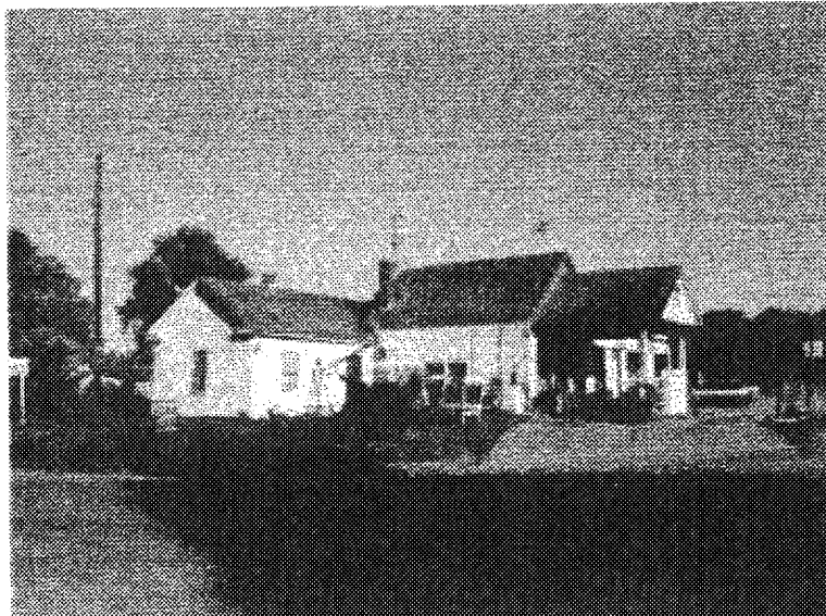
Figure 16: Harcum Store and Post Office (036-5013) Southwest corner
