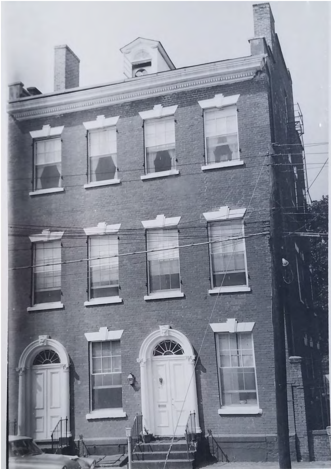
Figure 6 – On the right side of this circa 1960 photograph, the stone lintels of three windows on each floor can be seen, standing out against the dark brickwork. (“415 Prince Street,” n.d., Sommerville Photograph Collection, Alexandria Library, Special Collections)
