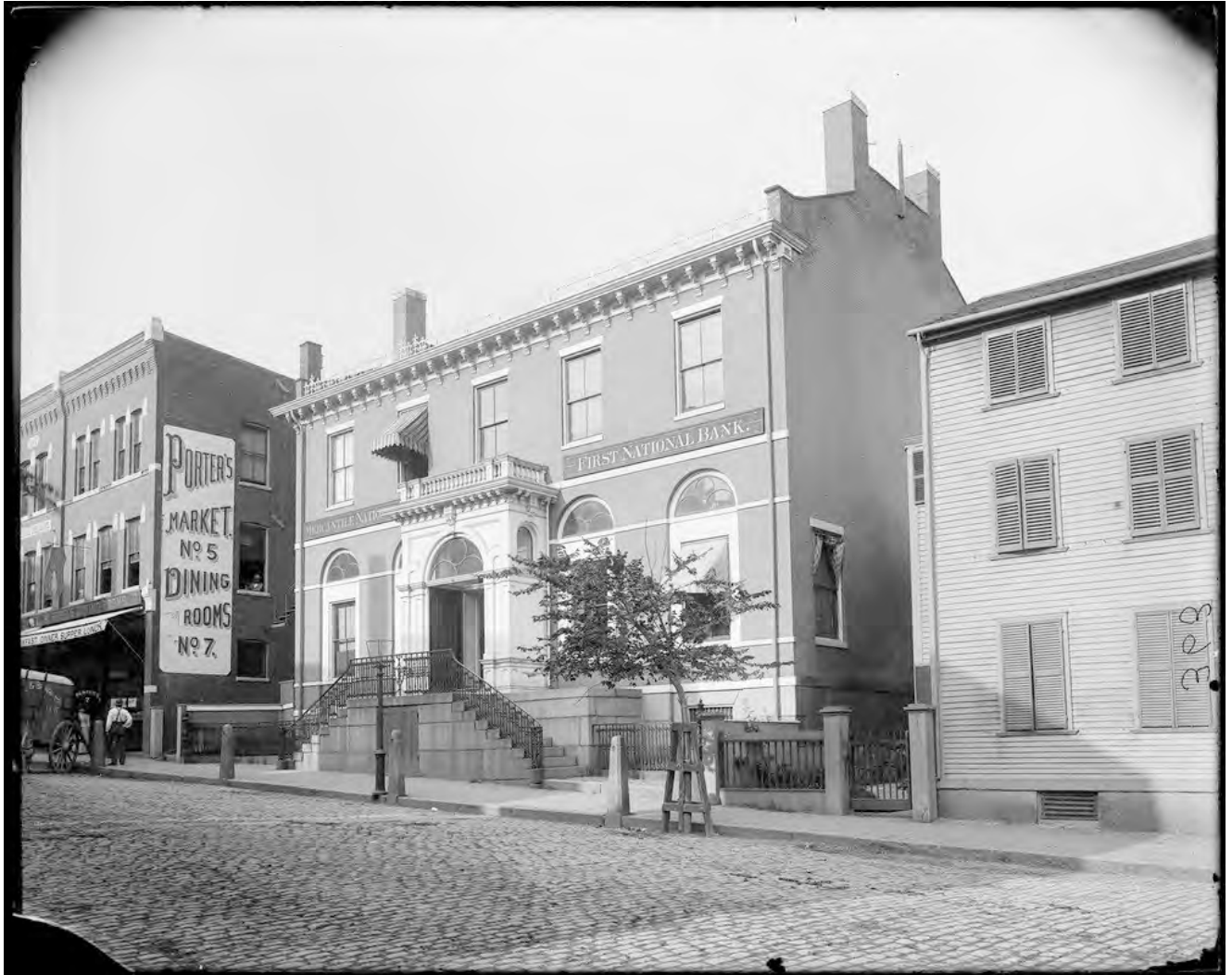
Figure 14 – Charles Bulfinch’s Essex Bank in Salem, Massachusetts (1811), displaying the tall, arched windows and planar exterior surfaces the architect frequently used. The portico is replacement of the original open, Ionic portico. (Frank Cousins, Digital Commonwealth [Massachusetts], ca. 1865-1914)
