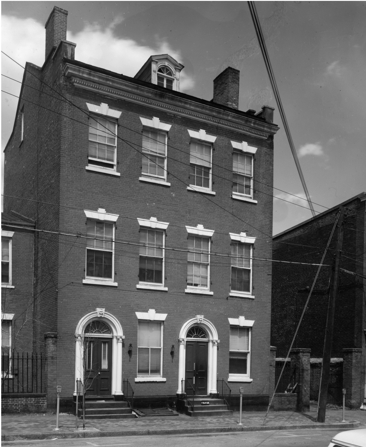
Figure 11 – This 1958 photograph shows glazed panels in the west door and one-over-one windows on the first floor of the original bank block, likely installed in the twentieth century. (Historic American Buildings Survey, Library of Congress)
