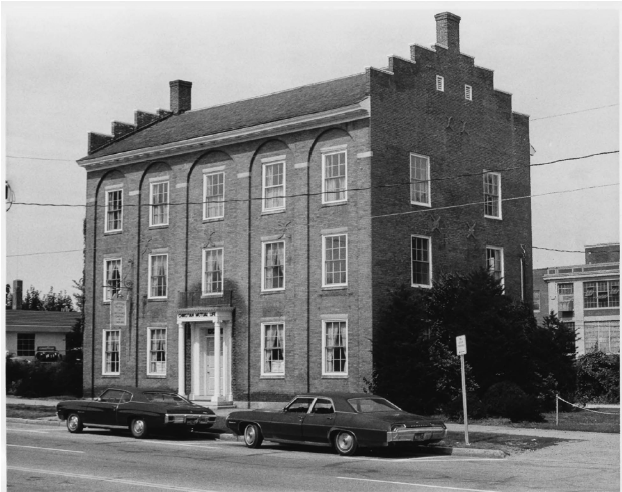
Figure 15 – Recessed arches capture the windows of John Leach’s 1826 bank building in Concord New Hampshire. (Merrimack County Bank National Register Nomination, 1979)
