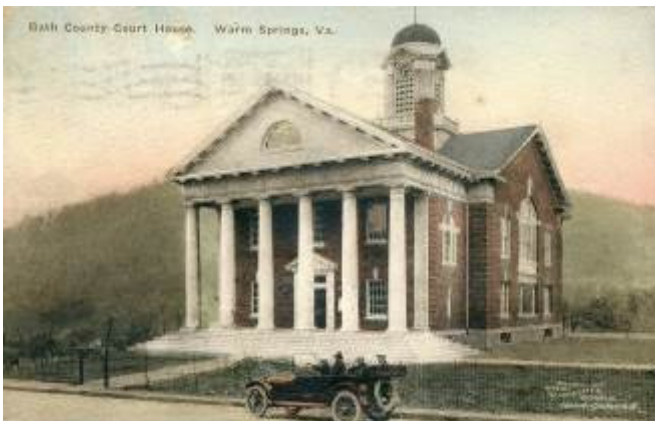
Ca. 1930c Post Card, Warm Springs Courthouse
