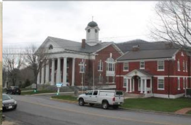
March 2017 Photo, Warm Springs Courthouse
