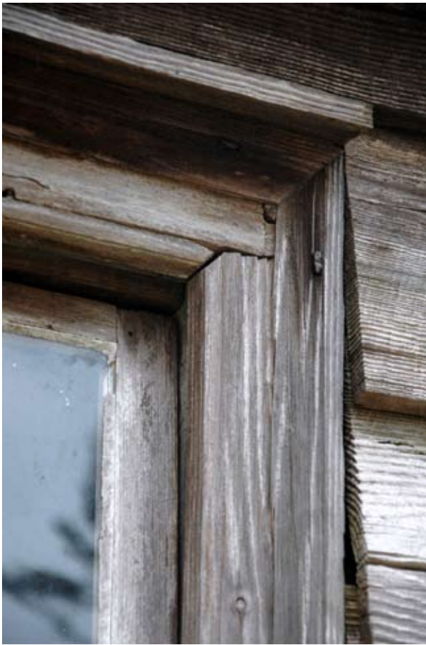
Figure 11. Original window frame.
