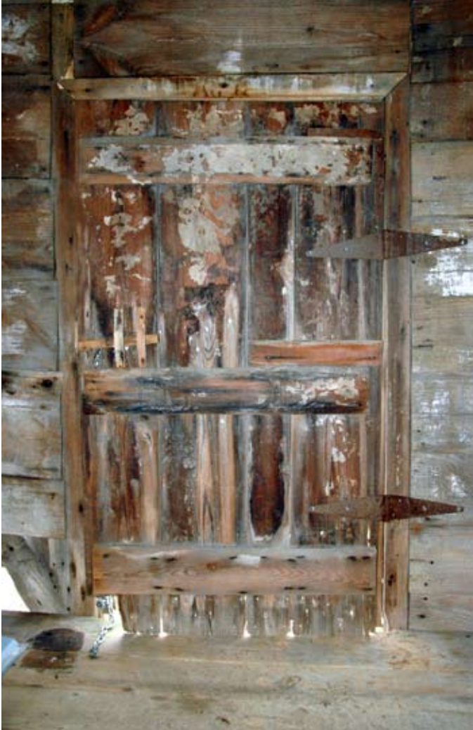
Figure 8. Interior of front door.
