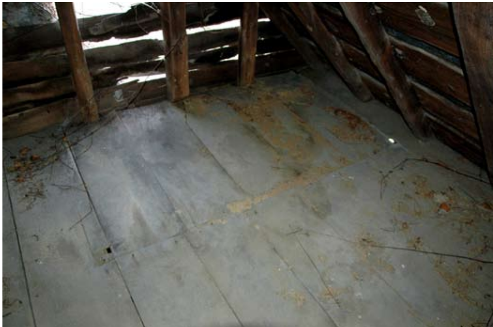
Figure 3. Closed stair opening and newel mortise.
