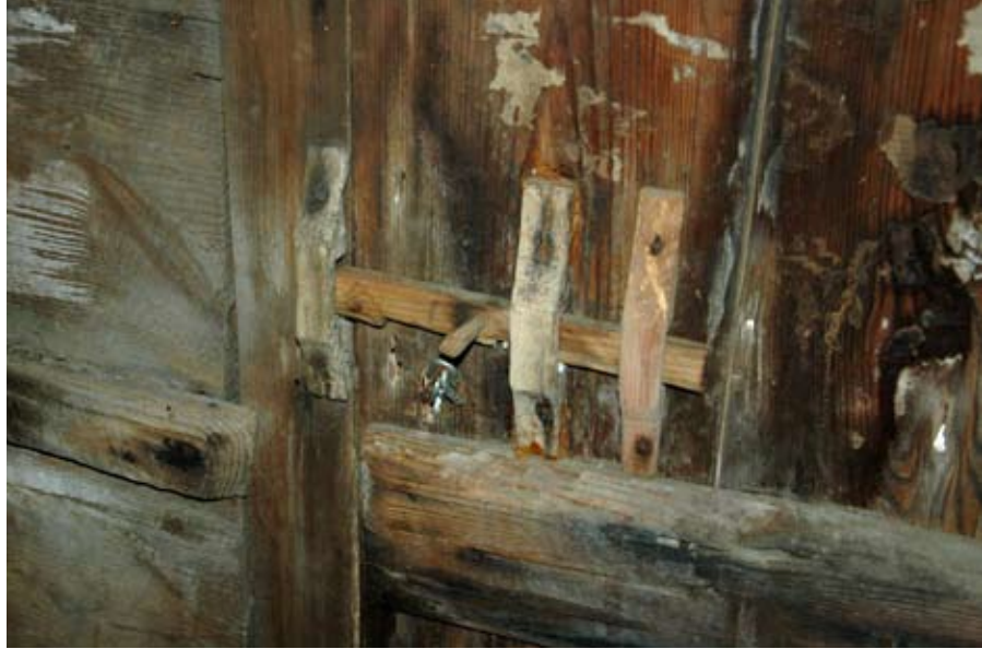
Figure 9. Original slide latch.
