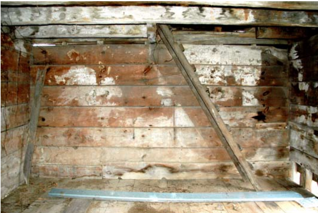
Figure 4. Nineteenth-century sheathing with ghost of Period II stair.
