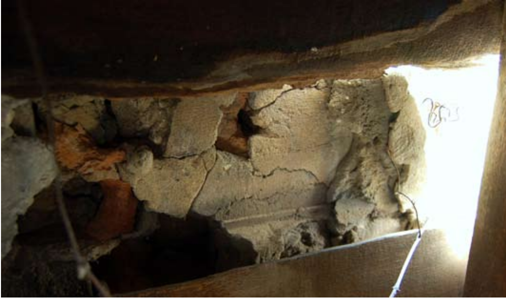
Figure 6. Mortar bearing impression of original, beaded weatherboard.
