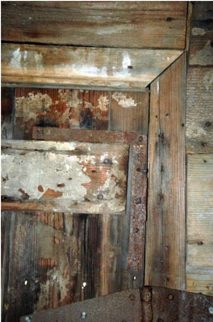
Figure 10. Remnant of original H-L hinge and head casing.
