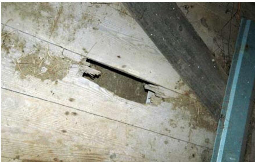
Figure 19. Failed flooring.
