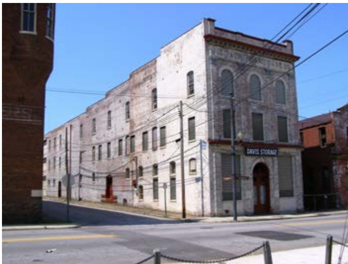
A commercial building in the Danville Tobacco Warehouse Historic District.
